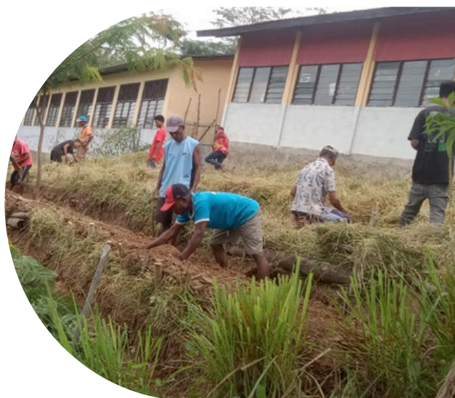
Terrace construction in Timor-Leste Permatil © Kiwa Initiative - 2024
